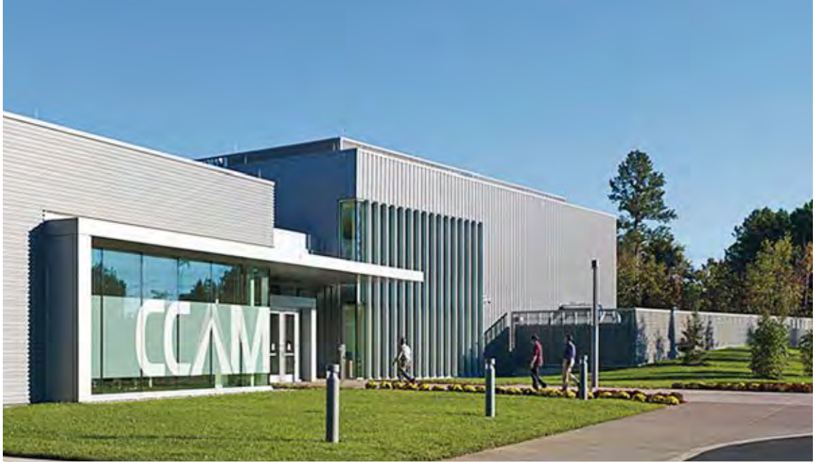
The Commonwealth Center for Advanced Manufacturing located in Prince George County, VA.
