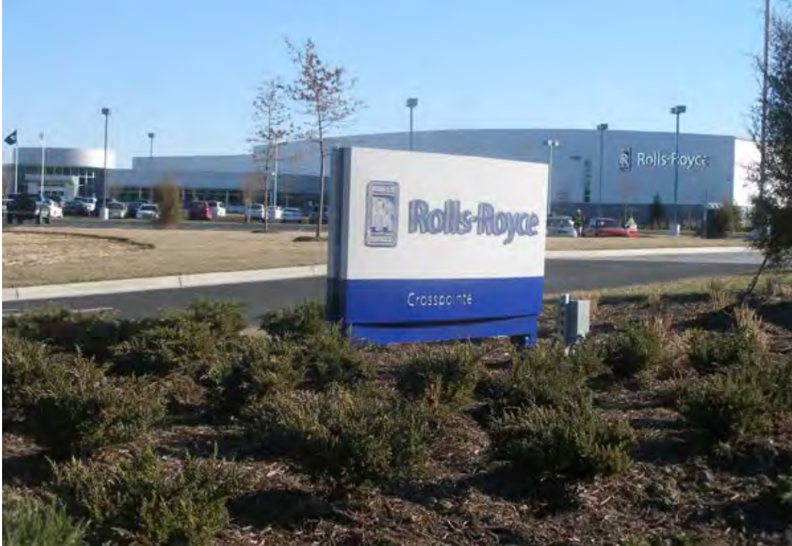
Rolls-Royce at Crosspointe Centre houses a research facility and several manufacturing buildings.
